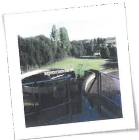
REHABILITATION DE LA STATION D'EPURATION
